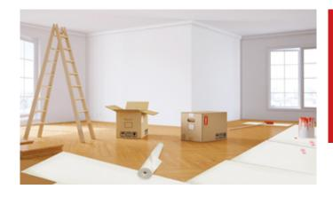
Isolmant Cover is installed with the non-slip side facing down and the transparent protective PE film facing up.
