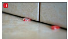
screed he is going to lay can "float" without establishing any rigid connection either with the load-bearing layers underneath or with the walls to its sides. Any uncovered points that could constitute an "acoustic bridge" must be covered with Isolmant Fascia Nastro.
