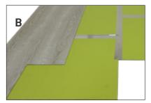
The flooring can be floating, taking care to lay it at an angle of 90 ° with respect to the underlay (Figure 2).
