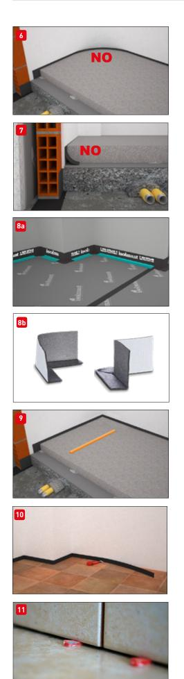
In conclusion, before proceeding with the laying of the finishing screed, the contractor must be reasonably certain that he has created a perfect watertight tank in which the cement screed he is going to lay can "float" without establishing any rigid connection either with the load-bearing layers underneath or with the walls to its sides. Any uncovered points that could constitute an "acoustic bridge" must be covered with Isolmant Fascia Nastro.
