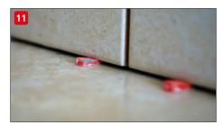
before proceeding with the laying of the finishing screed, the contractor must be reasonably certain that he has created a perfect watertight tank in which the cement screed he is going to lay can "float" without establishing any rigid connection either with the load-bearing layers underneath or with the walls to its sides. Any uncovered points that could constitute an "acoustic bridge" must be covered with Isolmant Fascia Nastro.
